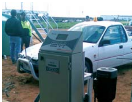
Control unit in front and fertigation tank in background (Lake Powell)
