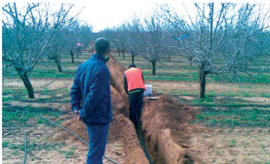
Installation of irrigation infrastructure at Lake Powell trial site
